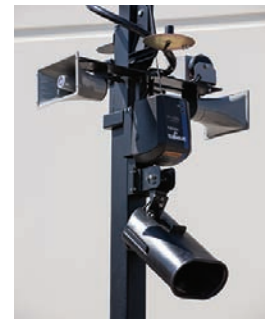
Public address system and license plate recognition (LPR) camera
